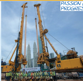
SUKE CB 3 & 4 – Construction of 303 nos of Bored Piles of various diameters of 1350mm to 3500mm for 4.5km elevated highway package.
