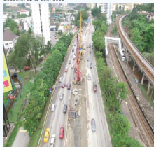
DUKE 3 – Construction of 9 nos. of Bored Pile of diameter 3500mm up to 50m deep
