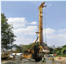
DASH CB 2 – Construction & completion of Bored Piling works of various diameters of 2000mm . 2200mm, 2500mm & 2800mm up to 68m deep
