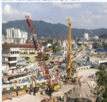
SUKE CB 3 & 4 – Construction of 303 nos of Bored Piles of various diameters of 1350mm to 3500mm for 4.5km elevated highway package.
